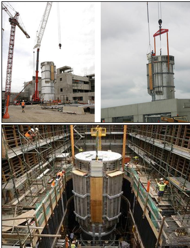
Installation of the OPAL Reactor Pool in 2004
