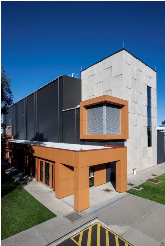
External view of the Synroc Waste Treatment Plant.
