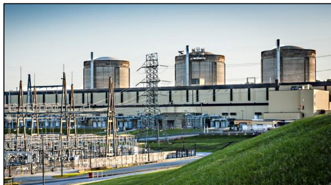
The three-unit Oconee nuclear power plant in South Carolina - three PWRs operating since the 1970s
