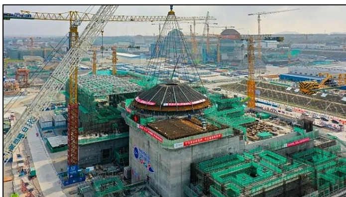
Dome being installed on Linglong One in China
