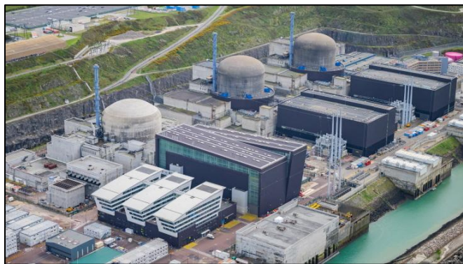
Flamanville 3 in foreground, Flamanville 2 and 1 in rear. (Image EDF)
