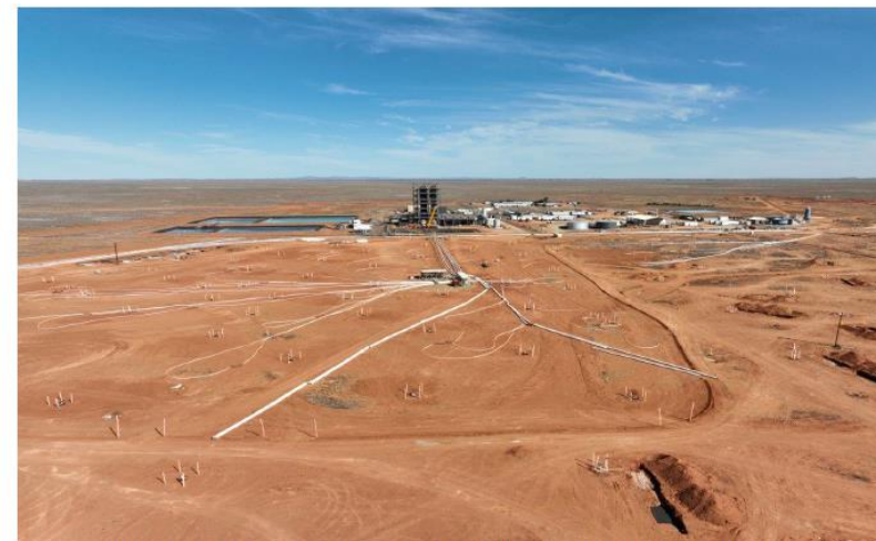
Image 1: Wellfield electrical, instrumentation, and piping materials has been installed
