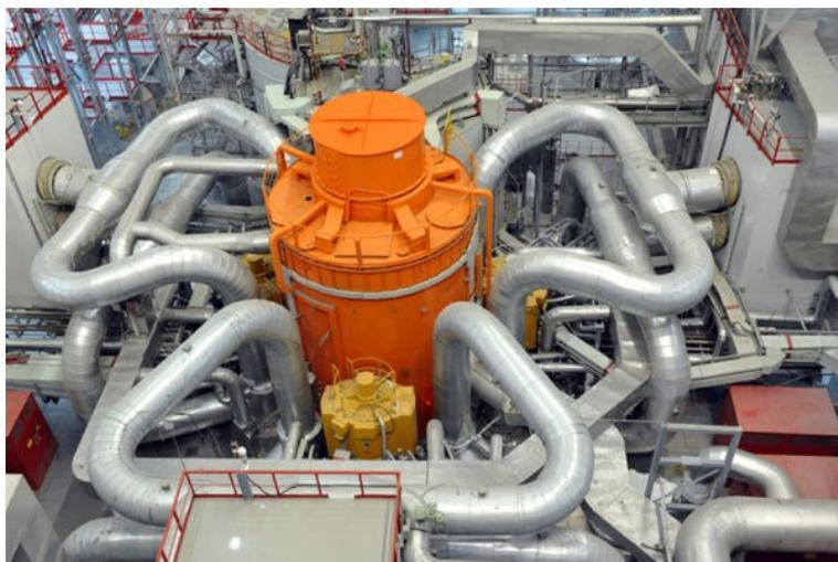
*Figure 2: BN800 sodium-cooled fast-neutron reactor in Russia*
