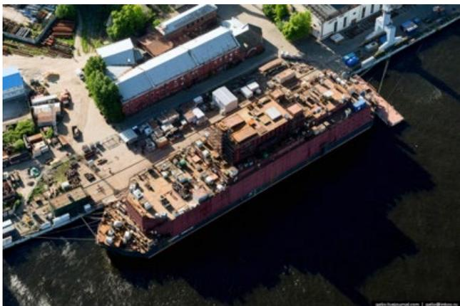
**Barge (140m long x 30m wide, 21,000 tonnes displacement) with 2 x 35 MWe SMRs under construction in St Petersburg. (Image courtesy of Rosatom)**
